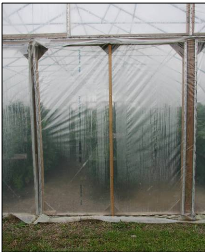
Figure 14. Peak-style high tunnel framing - close-up of end door.
