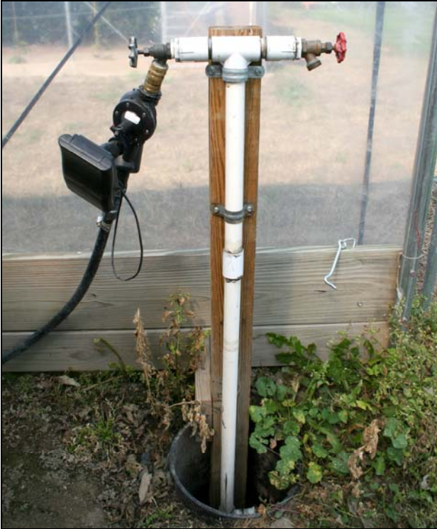
Figure 25. Drip irrigation ingress pipe with in-line water filter and faucet for hose attachment.
