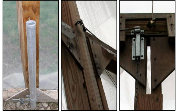
Figure 15. End door construction (L to R) door stop, pulley system for door closure, door closure.
