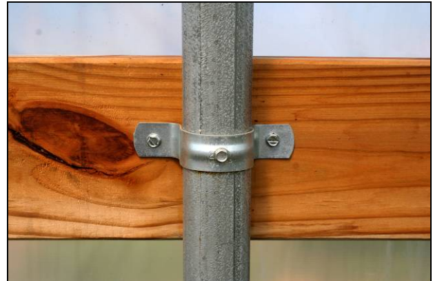
Figure 11. Peak-style high tunnel framing - side view showing close up of batten board fastening.
