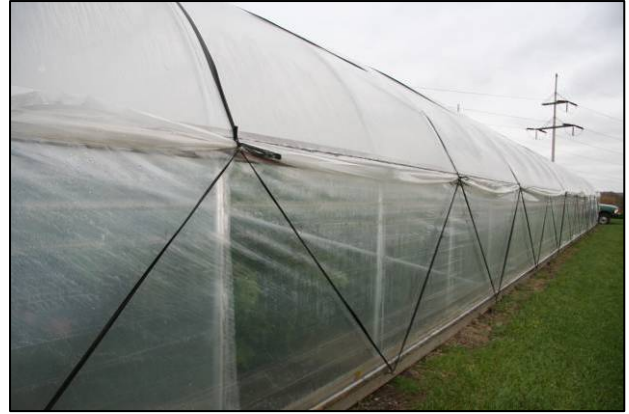
Figure 19. Webbing applied over plastic to keep it from blowing in the wind.
