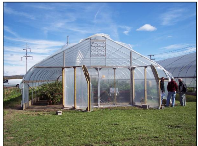
Figure 16. Hinged plastic covered tunnel doors.
