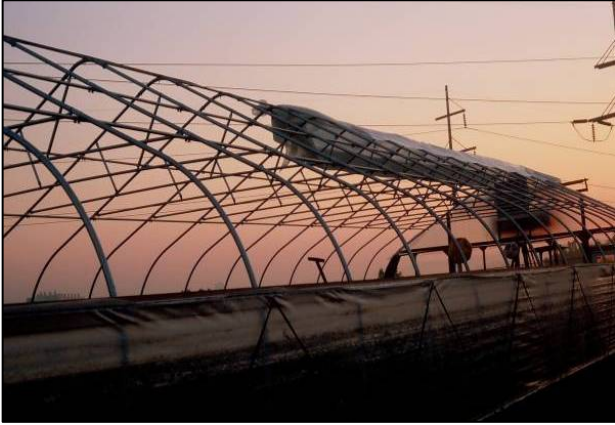
Figure 17. Applying the plastic over the high tunnel superstructure.
