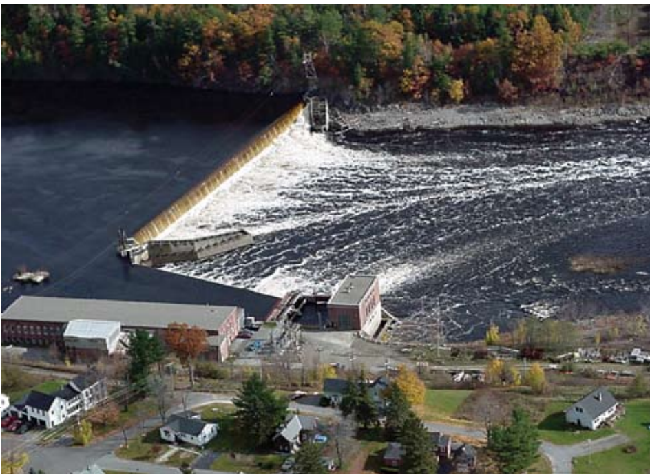
Veazie Dam, one of the dams to be removed to enhance fish passage.
