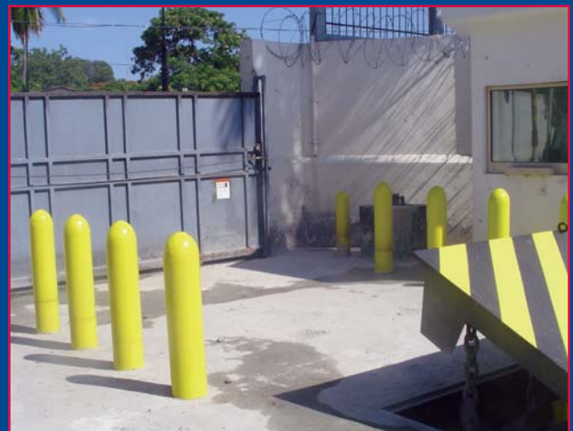
Perimeter gate with anti-ram bollards and vehicle barrier. PHOTO: USAID OFFICE OF SECURITY (SEC)
