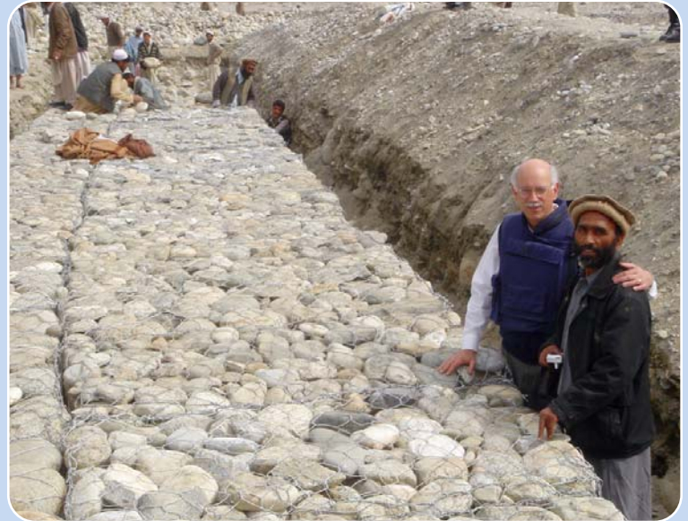
USAID Administrator Natsios with head engineer Askar in Muftie, Rodat (Nangarhar), Afghanistan. Building gabion walls and removing 25 years of built-up silt from the canals will significantly increase the flow of water to the affected area, enabling farmers to grow crops needing multiple floodings. PHOTO: USAID/MICHELLE PARKER
