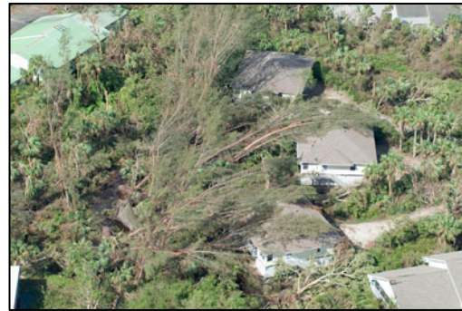
Figure 9-54. Fallen Australian pine trees cause extensive structural damage (Photo by SFWMD).
