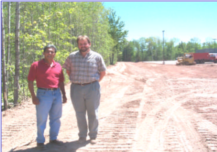
Luis Salas, NNAHA Injury Prevention Specialist and Dick Reese, NNAHA Environmental Health Officer photographed during the construction of the pedestrian/bicycle path
