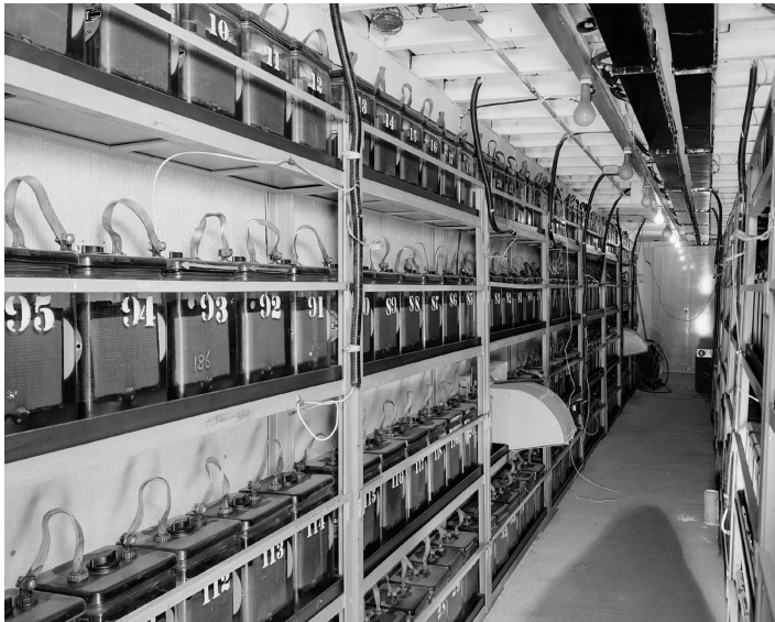
Fig. 2. Some of the batteries used to power the MANIAC I.
