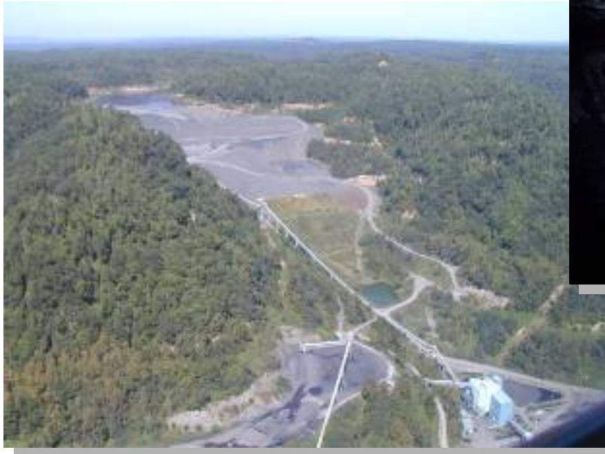
Prep Plant and Impoundment
