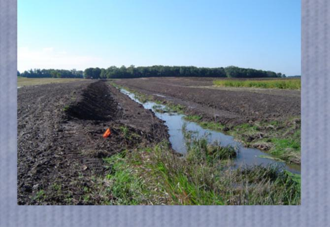
(Below) A mock overlay of the Michigan Ditch project, showing the existing ditch location and the constructed two-stage ditch. The image below shows the same cross section with the existing ditch data, the constructed two-stage ditch and the traditional ditch excavation. Notice the channel vegetation in the construction photo, the two-stage construction does not interfere with the channel or the vegetative growth.
