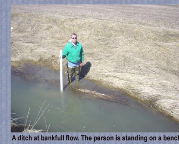
the infrequent flood events, there exists a dynamic equi librium where the amount of sediment imported is equal to that exported by the ditch system. Typically following construction or cleanout, benches will form within a few years and quickly reach a stable (neither aggrading nor
