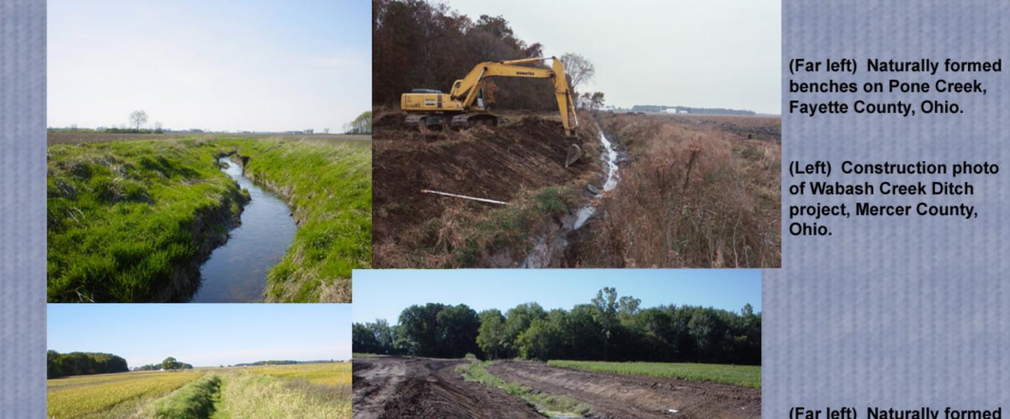
(Far left) Naturally formed benches on Loramie Ditch (Left) Constructed benches in Hillsdale
