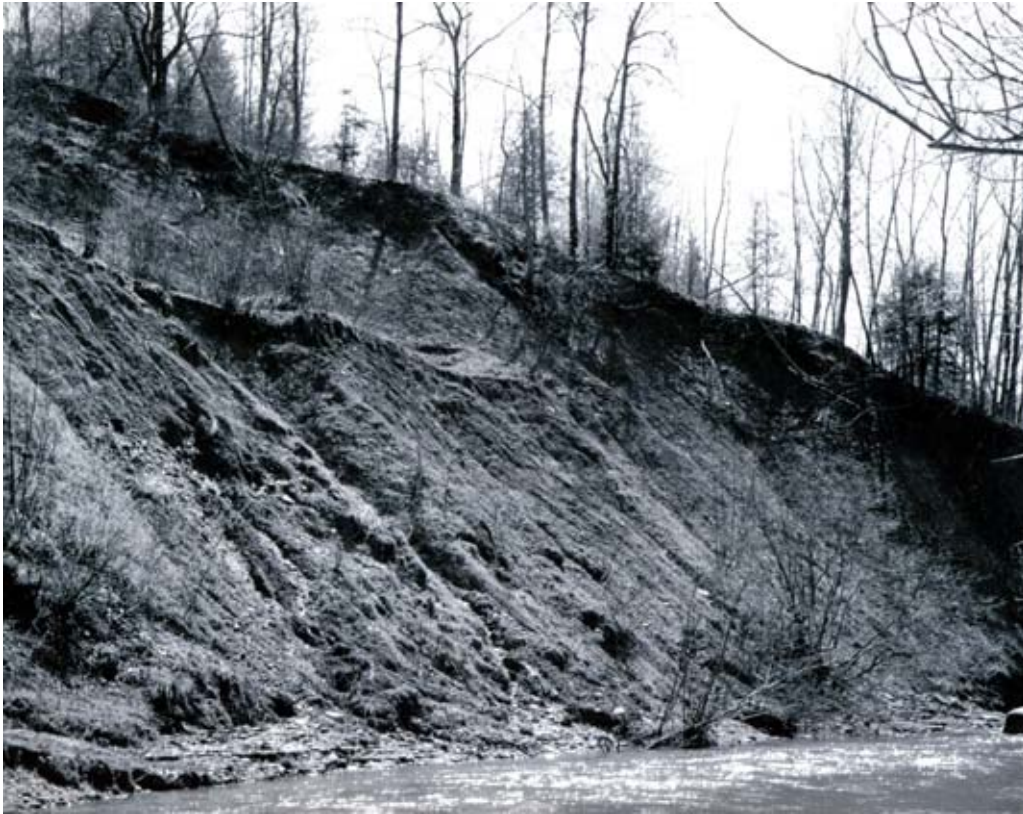
Figure 15.—Stream bank erosion on the bluffs of the South Branch of Cattaraugus Creek, in an area of the Rhinebeck-Hudson-Niagara general soil map unit.
