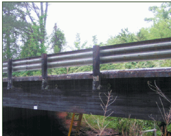
Figure 1. Transverse deck panels on glulam girders.
