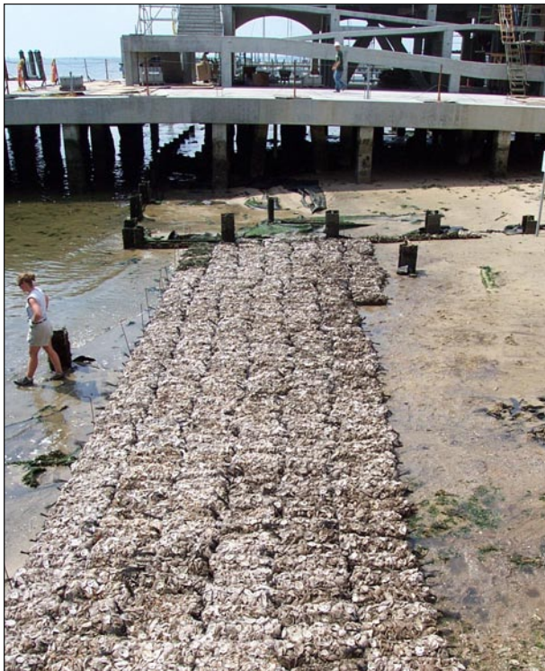
Figure 9. Volunteers place bags filled with oyster shells along the shoreline to form reefs. SCORE reef building project, South Carolina Aquarium. Photo courtesy of Loren Coen, Marine Resources Research Institute, South Carolina Department of Natural Resources.
