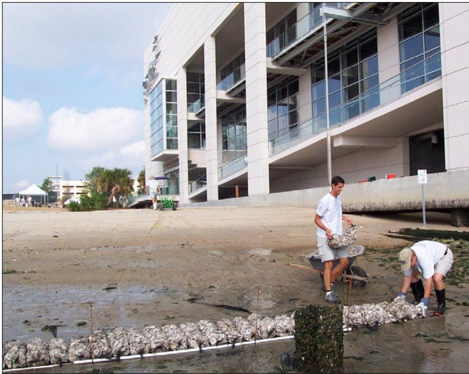
Figure 8. Volunteers use bags filled with recycled oyster shells to build large footprint reefs onto which oysters will settle, as part of South Carolina Oyster Restoration and Enhancement (SCORE) reef building project, South Carolina Aquarium. Photo courtesy of Loren Coen, Marine Resources Research Institute, South Carolina Department of Natural Resources.
