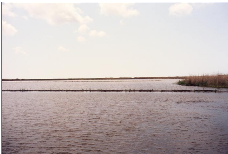
Figure 17. Two of the newly planted earthen terraces can be seen in the fore- and background of this photo. Terraces are only a few feet wide but that is sufficient to reduce wave energy and allow smooth cordgrass to become established, further reducing wave energy in the marsh. Photo by David H. Merkey, NOAA Great Lakes Environmental Research Laboratory.
