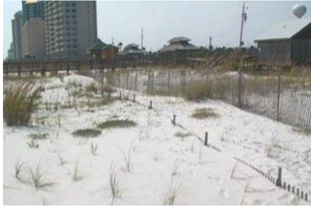
Primary and secondary sand fence.
