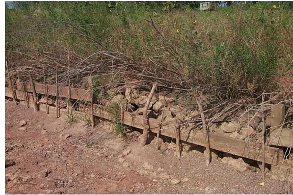
Constructed cribwalls planted with willow cuttings.
