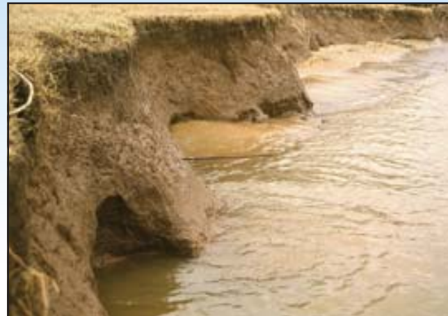
Typical eroding shoreline due to excessive wave action
