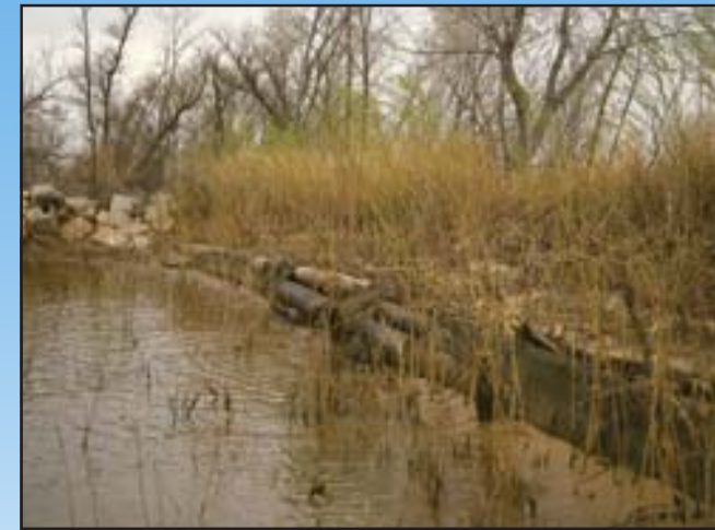
Log revetment technique for shoreline stabilization
