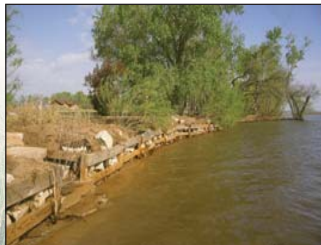
Cribwall technique for shoreline stabilization
