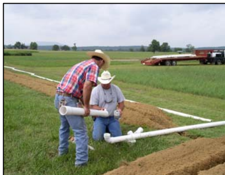
Installation of Irrigation System
