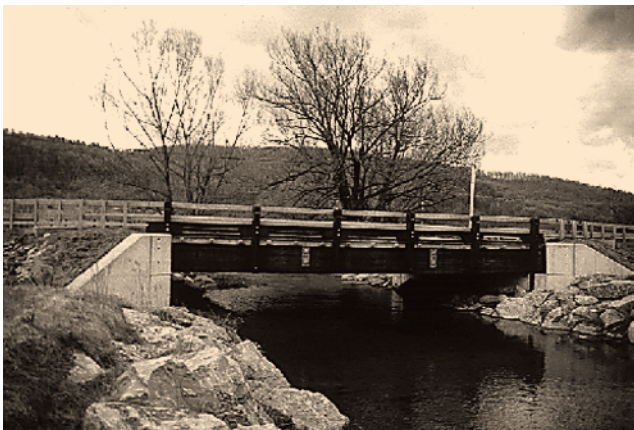
Figure 2—Typical bridge with stress-laminated deck.
