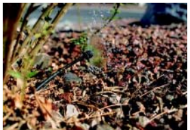
Low pressure sprinkler systems conserve water by delivering small amounts exactly where needed.
