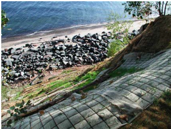
Stabilized slope with vegetative crib wall and slope grid
