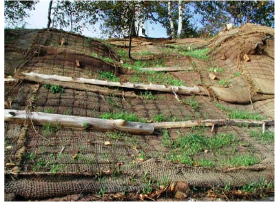
Vegetative crib wall and slope grid installed
