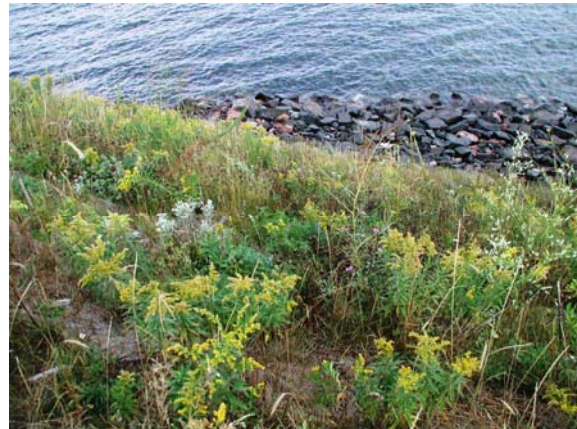
Fully stabilized and vegetated slope
