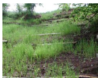
Establishing slope grid and vegetative cribwalls
