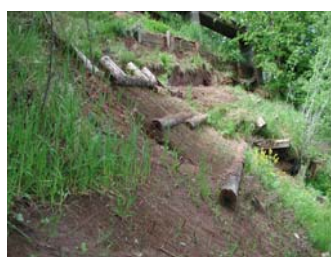
Establishing slope grid and vegetative cribwalls
