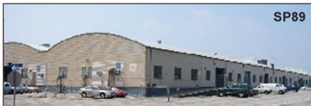
Figure 8—Primary types of buildings at NAVSTA Norfolk that contain wood: (top to bottom) conventional wood-framed construction (Facility A67), concrete and masonry with lumber framed and sheathed roof (A51), concrete and steel-framed with lumber-sheathed roof (LP4), and wood-framed walls and roofs with wood roof trusses (SP89).
