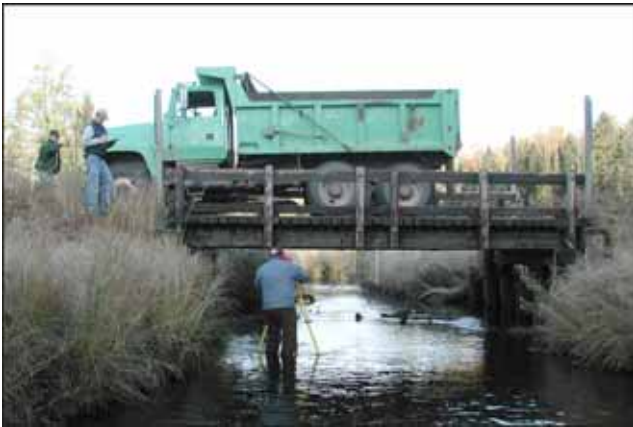
Figure 4—Static load testing of field bridges with fully loaded gravel truck.
