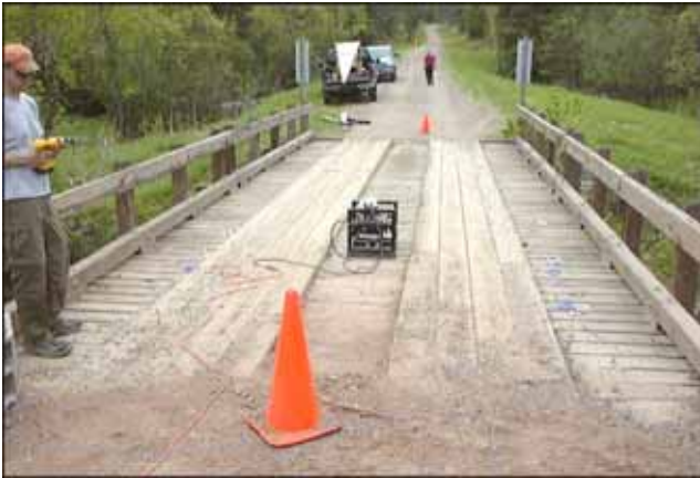
Figure 3—Forced vibration testing of field bridges with a forcing function.
