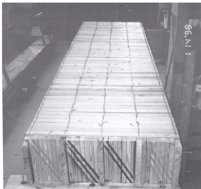
Figure 1. - Floor system under construction (top) and complete (bottom).
