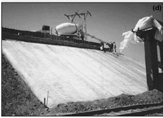
Figure 5—(a) Filter point mat, (b) uniform section mat, (c) articulated block mat, (d) concrete mat being used on a slope. (Used by permission: copyright Elish Construction, Inc.)
