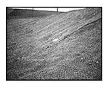
Figure 1—Coconut fiber mats. (Used by permission: left and center photos, copyright Aspinwall Group; right photo, copyright Hy-Tex.)
