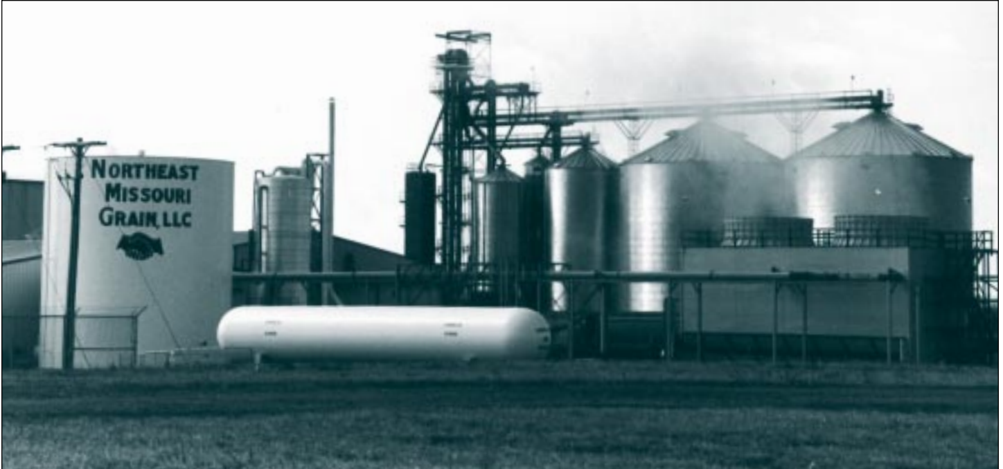
Corn growers formed a value-added cooperative to build this ethanol plant in Northeast Missouri.
