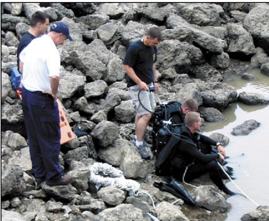
Portland District Dive Safety Officer Rick Benoit (in white) and four of his divers work below the dam at Elk City Lake during a stilling basin inspection. (Photo provided by Tulsa District.)
