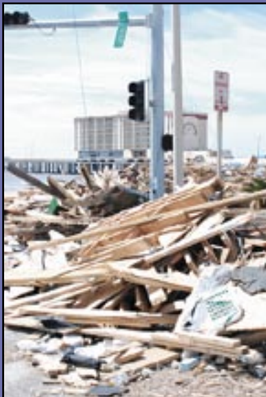
This is a minute portion of the damage dealt by Hurricane Ike as it swept through Texas. (U.S. Army Corps of Engineers photo.)
