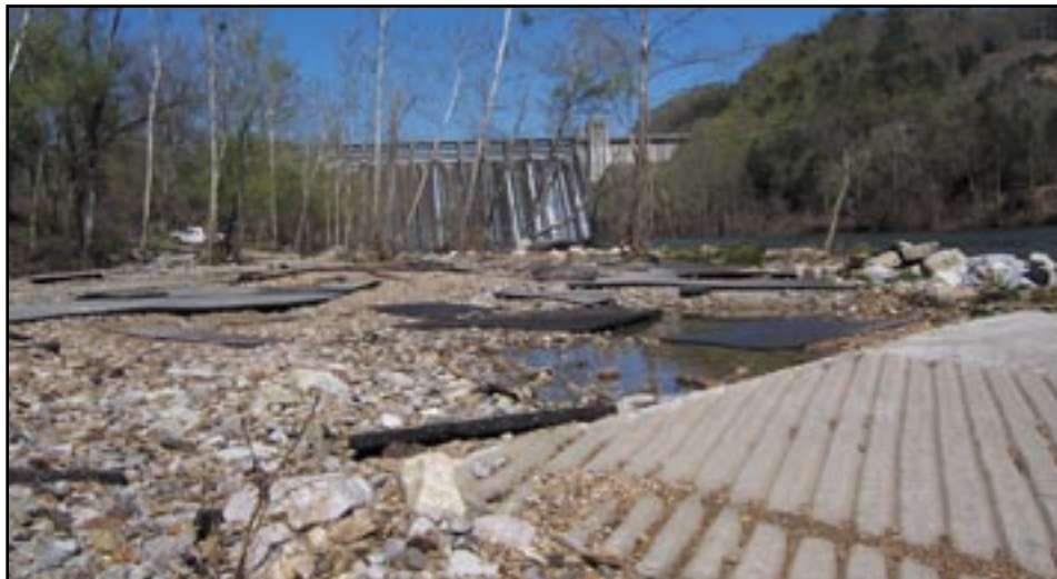
This flood-damaged public access area below Norfolk Dam is one area where a Damage Survey Report is applicable. One was prepared to determine repairs required to bring the area back to pre-disaster condition. (Photo provided by Little Rock District.)
