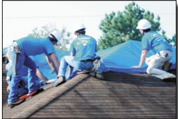
Contractors working for the U.S. Army Corps of Engineers install FEMA Blue Roofs on houses damaged after Hurricane Ike ripped through Texas. The Corps manages Operation Blue Roof for FEMA after disasters like Ike. (USACE photos.)
