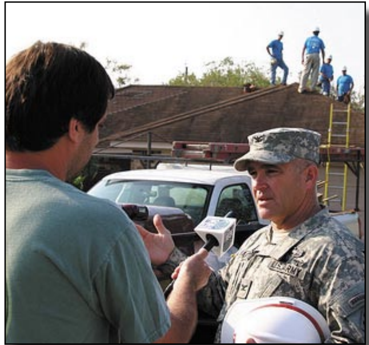
Col. Christopher W. Martin, U.S. Army Corps of Engineers Fort Worth district commander, talks to local media in south Houston at the site of the first Operation Blue Roof installation following Hurricane Ike. Martin, commander of the Task Force Pacesetters recovery field office in Pasadena, Texas, was working to spread the word about Operation Blue Roof. (U.S. Army Corps of Engineers photo.)
