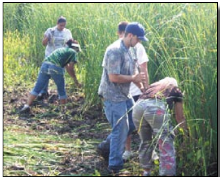
Approximately 60 volunteers turned out at Waco Lake on Saturday, Sept. 27th, to celebrate National Public Lands Day. They performed a variety of tasks, but at the Waco Wetlands they reinforced a concrete embankment and removed invasive cattail vegetation.
