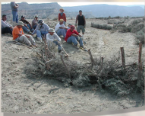
Jemez Pueblo ranchers constructed a series of post and wicker weirs using locally available juniper branches and sagebrush.
