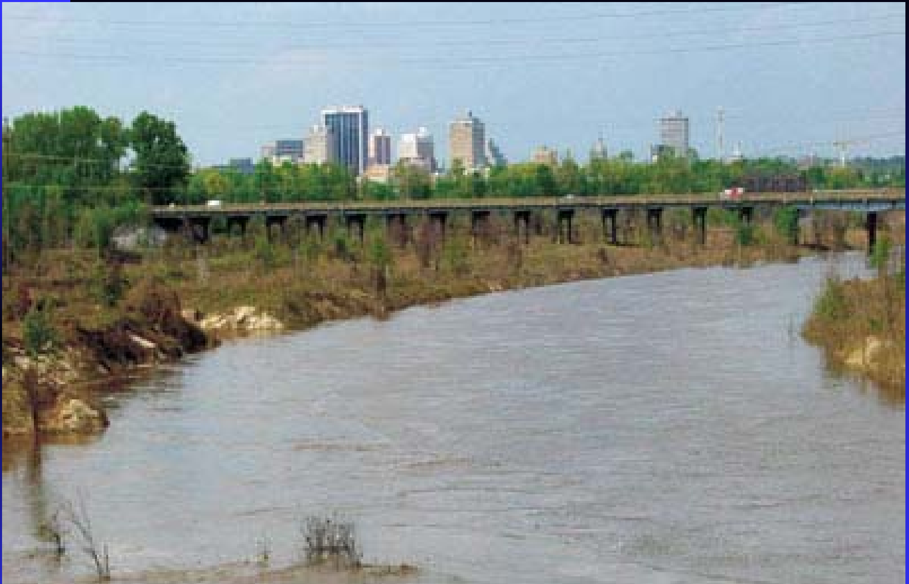
Figure 5: A View of Pearl River Across HYW 55 In The City of Jackson and The Threats of Urban Land Use
