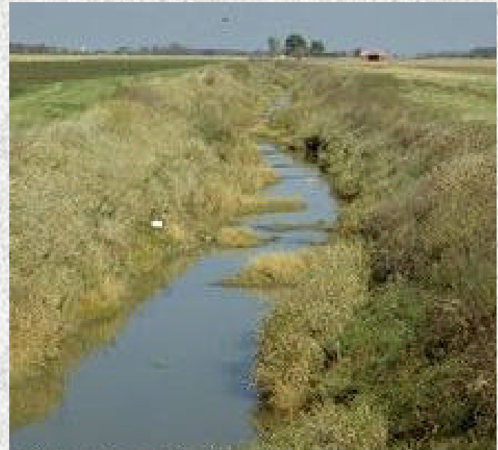
Stream channelization. (Photo: US EPA)
