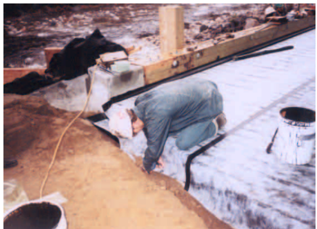
Figure 13—Installation of waterproof membrane.
