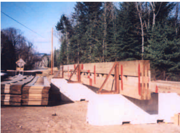
Figure 8—Preassembly of laminations into mini-modules at bridge site.
