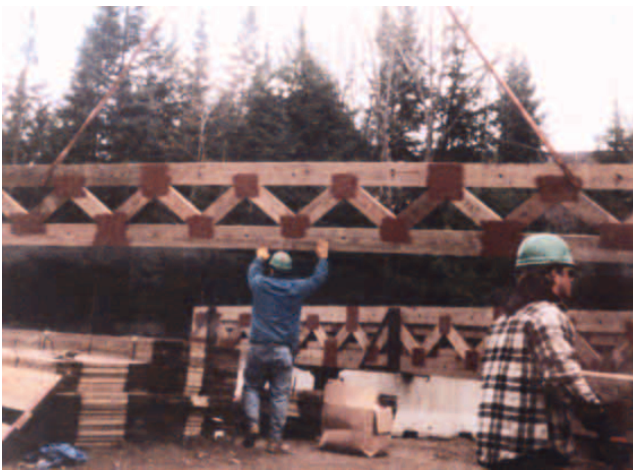
Figure 7—Placement of painted trusses onto temporary supports for formation of mini-modules.
