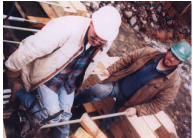
Figure 10—Tightening of stressing bars during stressing.
