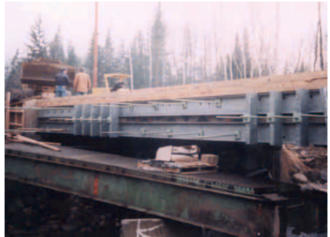
Figure 9—Installation of stressing system.
