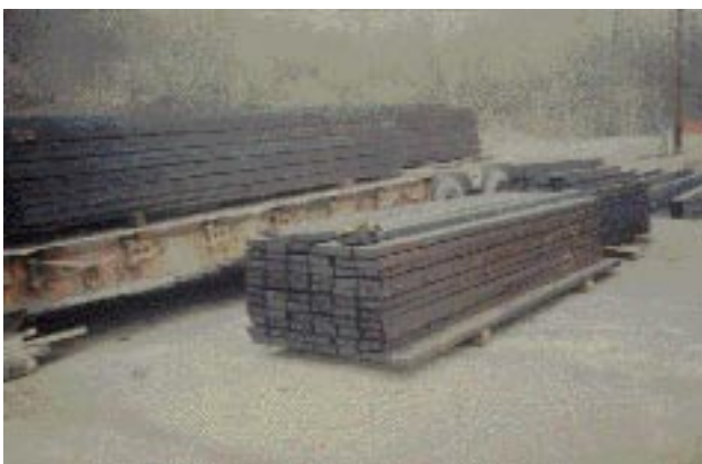
Figure 7—Delivery of timber components to the bridge site with tractor trailers.
