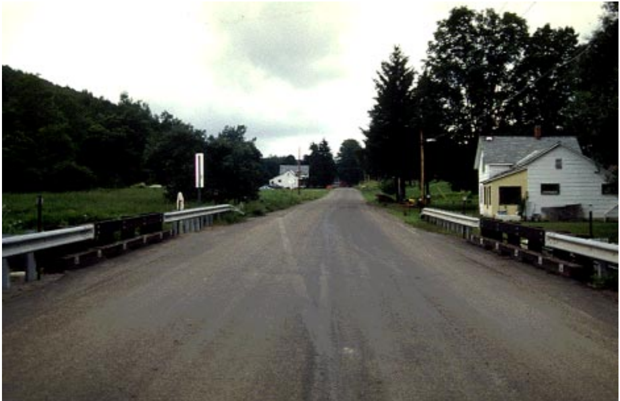
Figure 10—Completed Christian Hollow bridge: (top) side view, looking Northwest; (bottom) end view, looking west.
