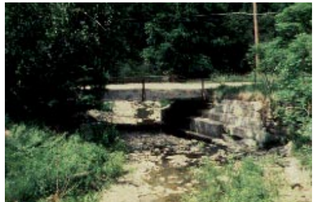
Figure 2—Original bridge constructed in the 1950s.
