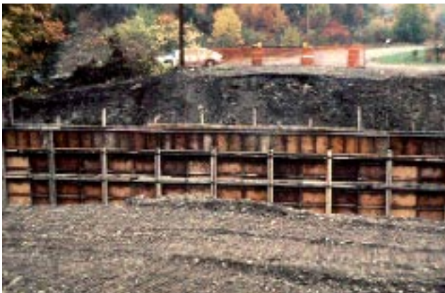
Figure 6—Construction of reinforced concrete abutments.
