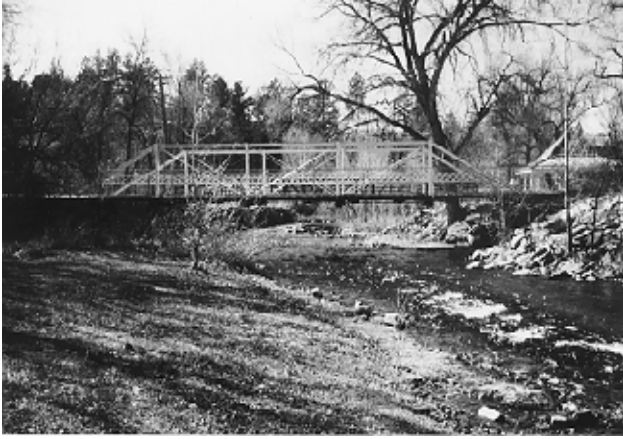
Figure 2—Original Spearfish Creek bridge constructed in the early 1950s.
