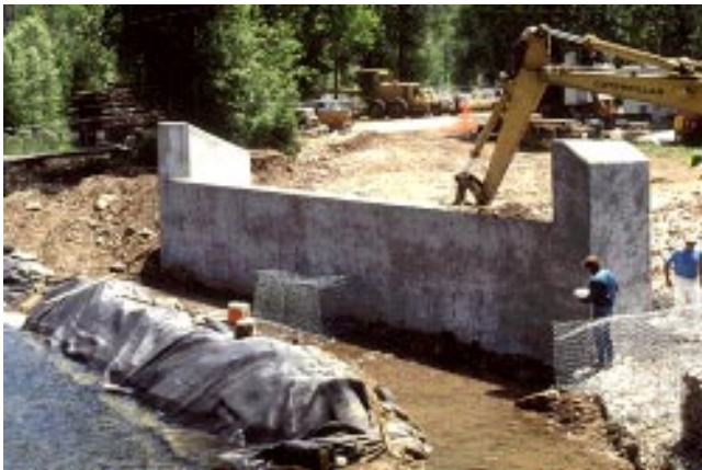
Figure 6—Construction of reinforced concrete abutments and wingwalls.
