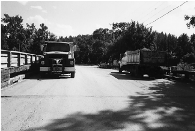
Figure 16—Load test 2 truck positions for load cases 3 and 6 (looking south).
