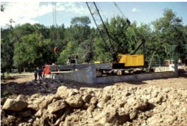
Figure 10—Lifting preassembled bridge modules onto concrete abutments with an overhead crane.
