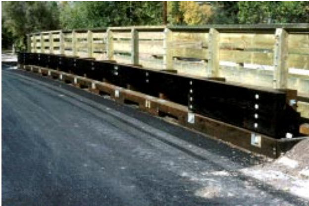
Figure 12—The completed rail system and pedestrian sidewalk.
