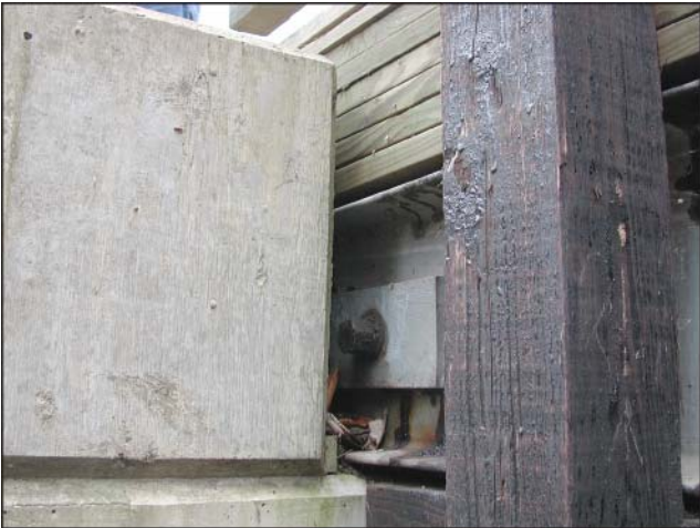
Figure 18—Concrete abutment “cheek-wall,” which prevents access to end bars for re-tensioning.
