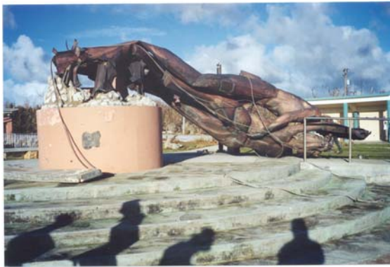
Figure 20. (a) Toppled statue at Two Lover's Point. Note failure of guy wires. (b) Severely damaged wood-rotted and termite-infested wooden house in Maite. (NOAA Photos)
