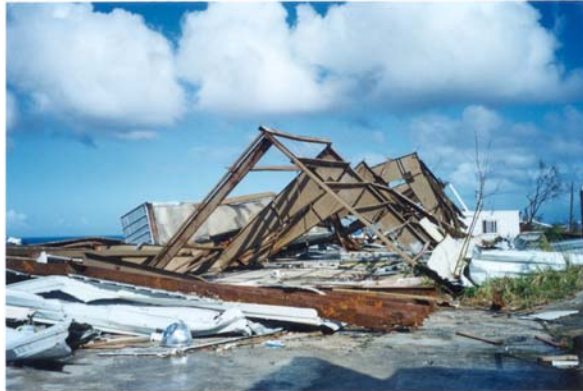
Figure 23. (a) Industrial building near the cliff line at Maite. (b) Same building from another angle. Note overturned container that may have helped to destroy the building. (NOAA Photos)
