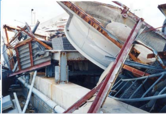
Figure 19. (a) Severely damaged typhoon doors of a major Upper Tumon hotel. (b) Severely rusted and corroded frame and connectors of one of the air conditioning units at a major Upper Tumon hotel.
