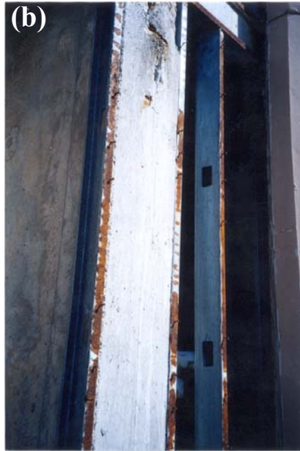
Figure 17. (a) A major hotel in Lower Tumon. Note the in-tack doors leading to the balconies. (b) Missing lightweight exterior wall panels of a lower Tumon hotel, with very small rusted attachment points of connectors and the appearance of glue residue. (NOAA Photos).
