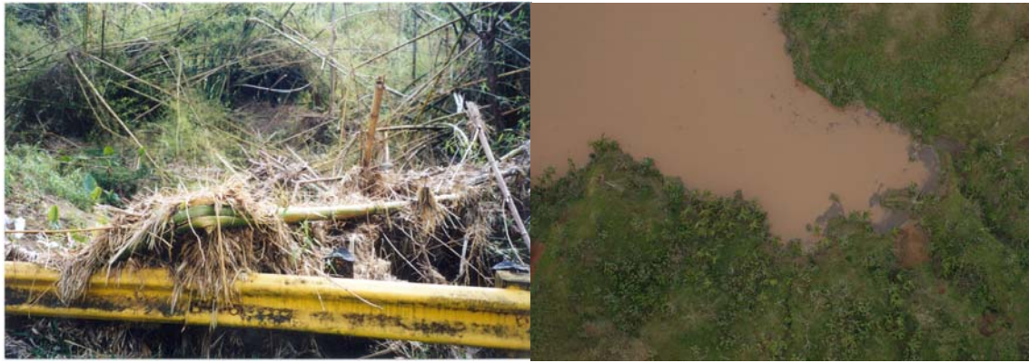
Figure 26. (a) Erosion and debris accumulation at a bridge, due to record rainfalls in central parts of Guam. (NOAA Photo) (b) Silt and debris in the Fena Reservoir on the US Naval Magazine following Typhoon Pongsona. (Official Navy Photos by JO1 Melody Kight Courtesy of COMNAVMAR)
