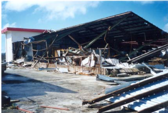
Figure 23. (a) Industrial building near the cliff line at Maite. (b) Same building from another angle. Note overturned container that may have helped to destroy the building. (NOAA Photos)
