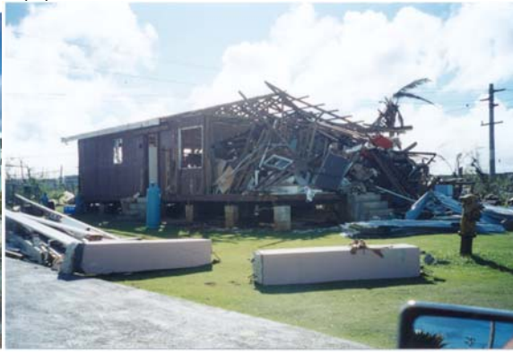
Figure 20. (a) Toppled statue at Two Lover's Point. Note failure of guy wires. (b) Severely damaged wood-rotted and termite-infested wooden house in Maite. (NOAA Photos)
