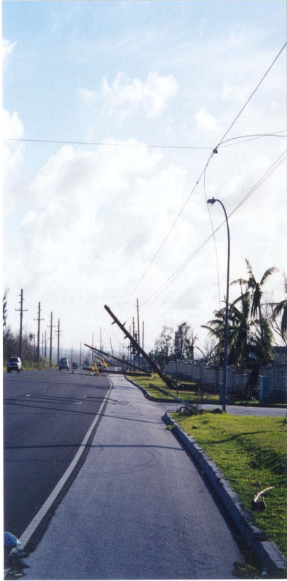
Figure 25. (a) Damage to hollow-spun concrete power poles at Carnation Road in Latte Heights, Dededo. (b) Some hollow-spun concrete power poles were improperly constructed with the pre-stressing steel cables bundled down the hollow center instead of being imbedded in the concrete. (NOAA Photos)
