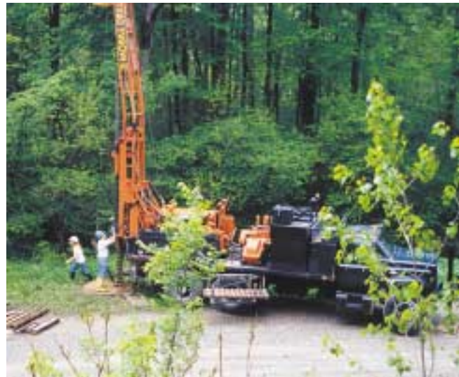
Drilling a well to tap groundwater.
