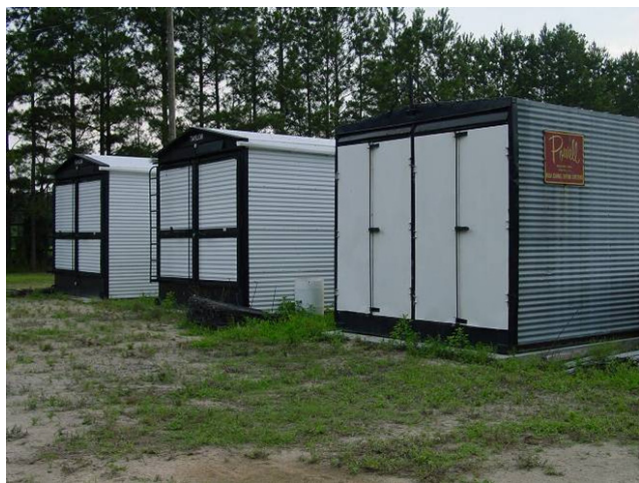
Fig. 8. Flue-cured tobacco kilns in eastern North Carolina.
