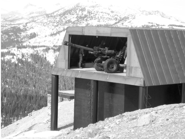
Figure 10: 105 Howitzer inside a protective shelter.
