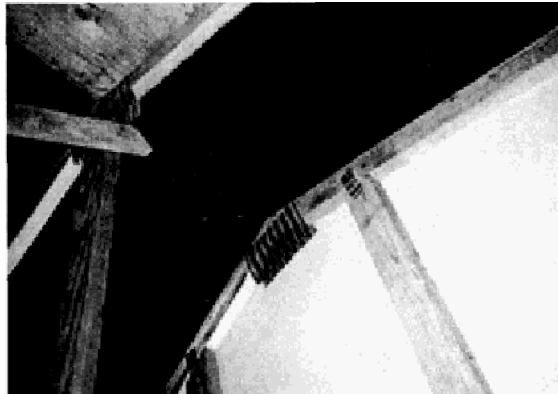
Figure 1. Inside view of failed FRT plywood roof sheathing.
