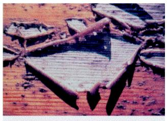
Film-forming finishes aren't good for decks. Paints, varnishes and other finishes that form solid films are bad for use on decks because of exposure to sunlight and moisture cycling.
