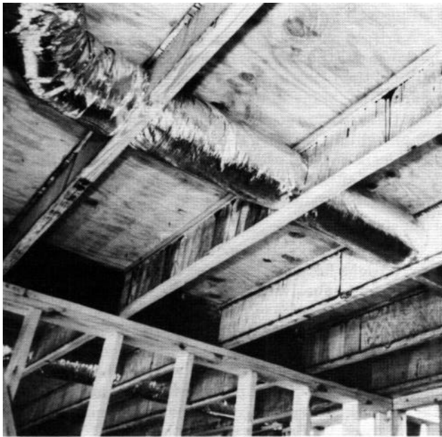
Figure 4. – Wood I-joint floor system (a) allowing passage of large ducts through the web, and (b) including hangers for connection to glued laminated beam.
