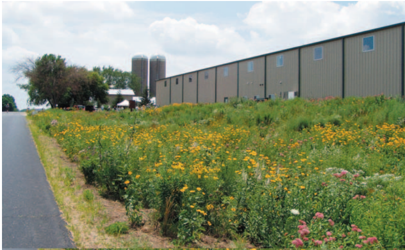
The seed cleaning building at Agrecol's Rock Prairie Farm, Evansville, Wisconsin. This building is heated with their own native grass biomass pellets.
