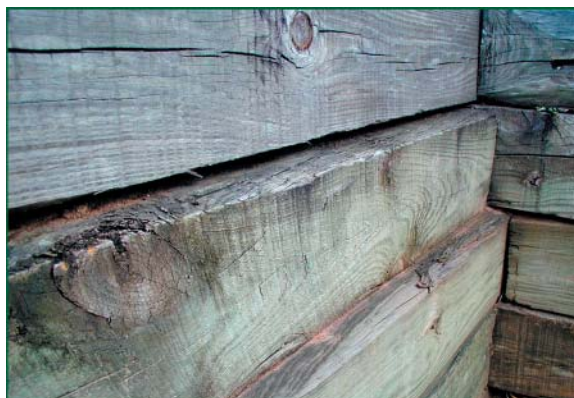
Residential retaining wall fabricated from treated (green) timbers.
