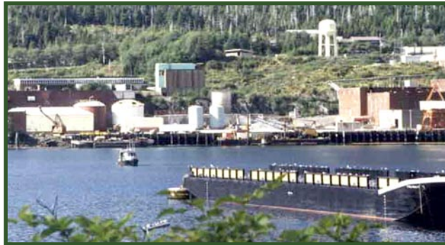
Thermal degradation is of concern in industrial buildings.
