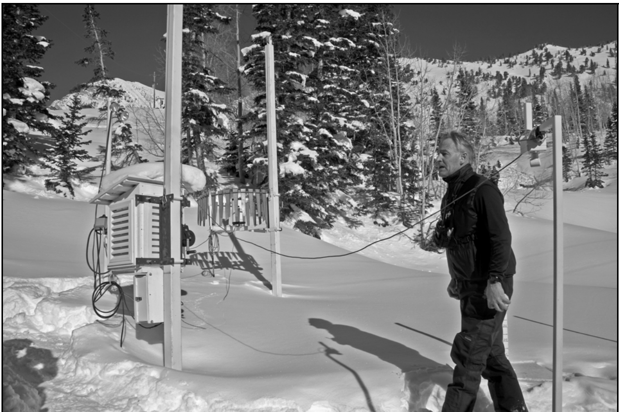
Figure D.1 The Utah Department of Transportation's study site in Alta, Utah (photograph by Bruce Tremper).
