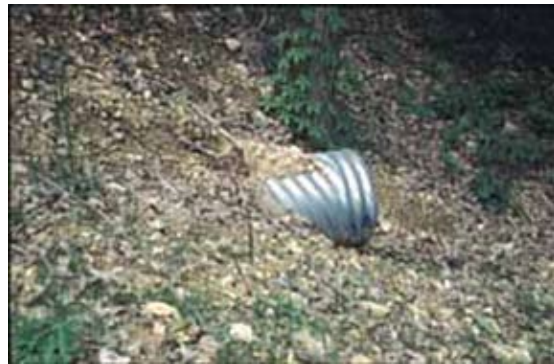
Culverts transfer water under a road, reducing soil erosion.
