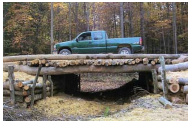
Bridge constructed with on-the-farm materials.
