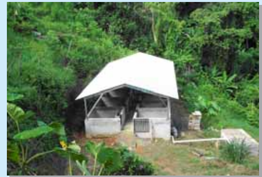
Demonstration animal waste management facility at a small swine operation in Rio Piedras, Puerto Rico
