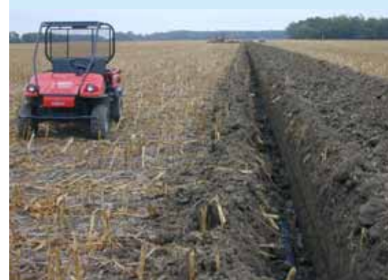
A new tile drain in northeastern Ohio.
