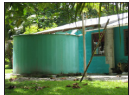
A typical rainwater catchment tank
