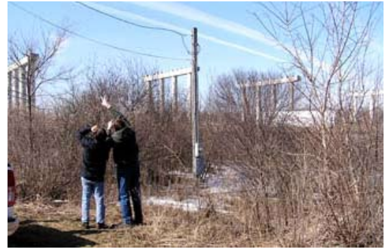
Zhining Tao and Kent McClure evaluate a potential road salt sampling site along the Chicago I&M Canal. In the background are bridge supports for the 12.5-mile I-355 south extension project. The project is part of the Illinois Toll Highway Authority's $5.3 billion Congestion-Relief Program to reduce travel times.
