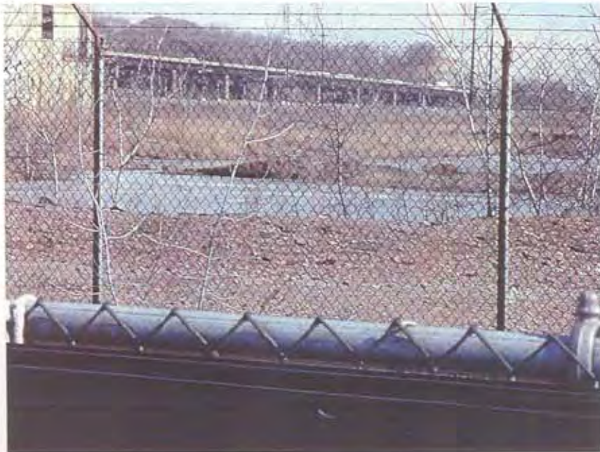
Photograph 4: The lagoon system
