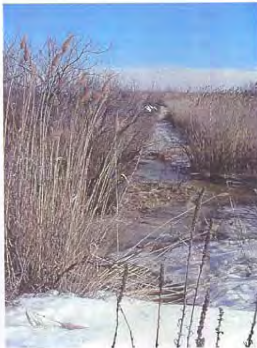
Photograph 6: The southern drainage ditch
