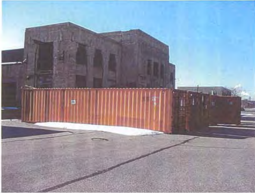
Photograph 7: Sea boxes containing dioxin-contaminated asbestos among other process wastes
