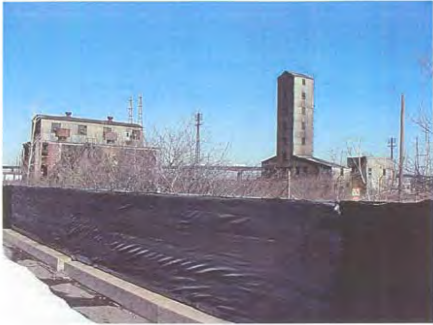
Photograph 3: The former distillation building in the lagoon system area
