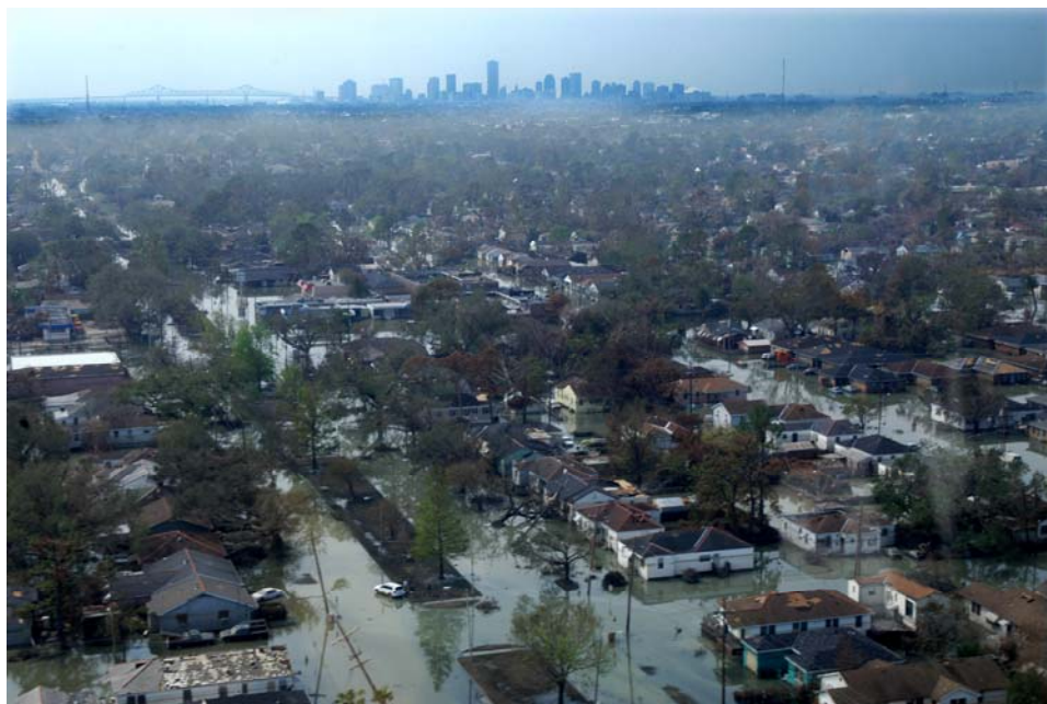
Figure 2-1. New Orleans was inundated by floodwaters following Hurricane Katrina.
